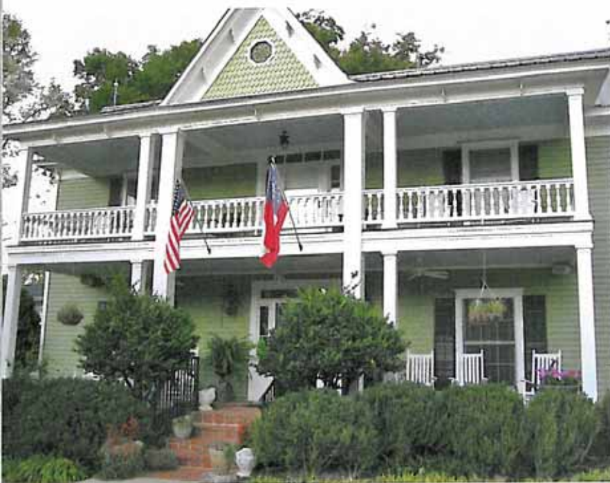
Rush and Sharon Mauney saved their late-19th-century, north Georgia home from destruction in a fire drill.
